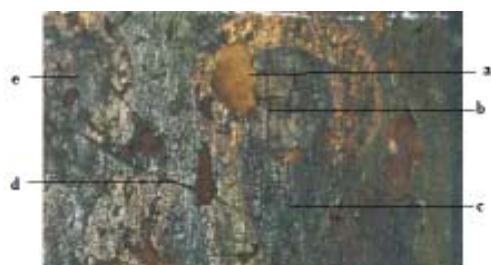
Fig. 3. Deterioration of the painting layer: a – deep gaps; b – old age rough cracks; c – old age fine cracks; d- scratch; e - clogged dirt;
